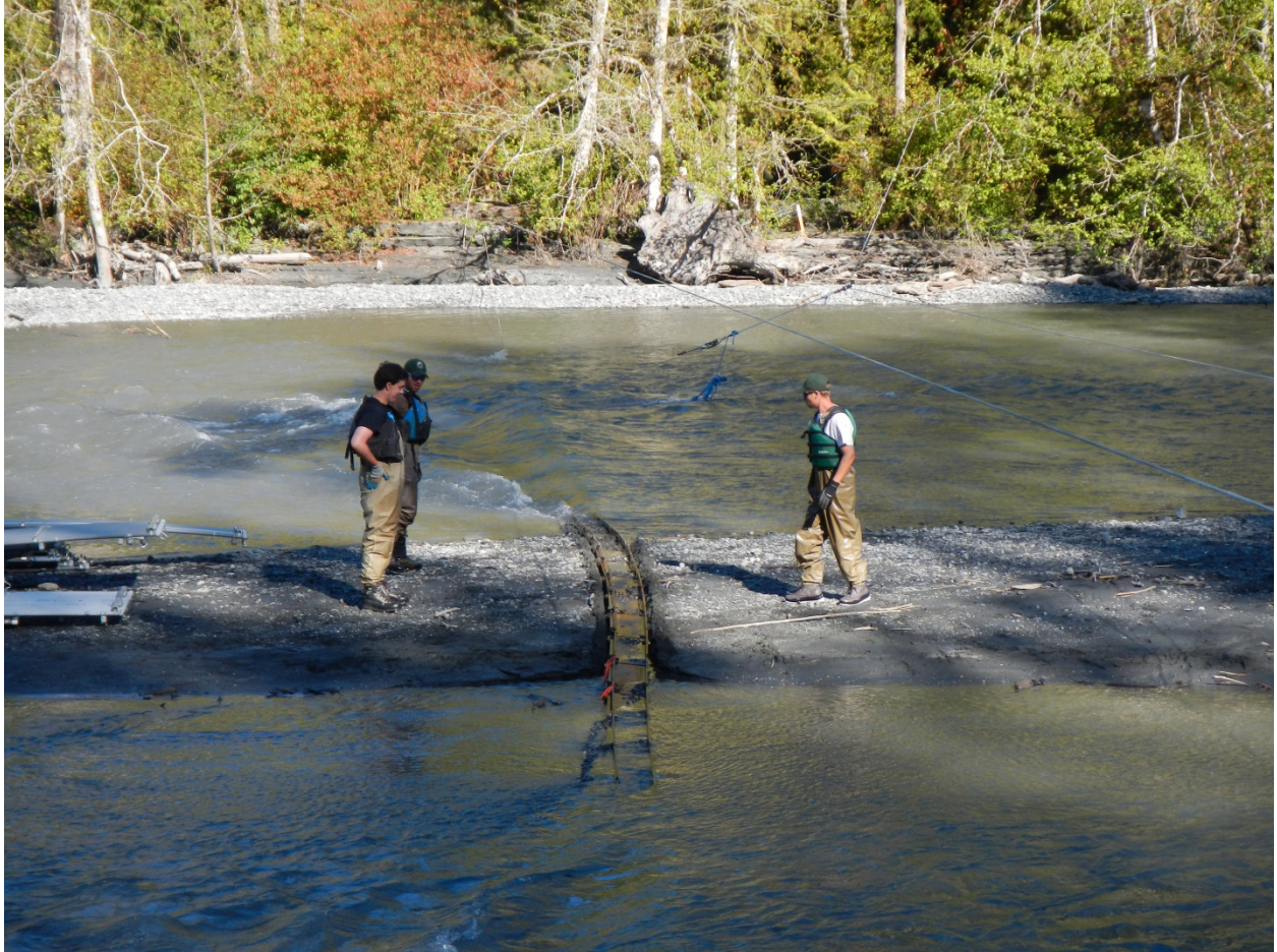
Figure 1. Newly designed, channel conforming substrate rail exposed on central gravel bar, looking from left bank channel across to right bank channel. Photo taken July 24 2013, discharge = 1,050 cfs (USGS gage 12045500).
